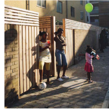
1. - 1.8m high brick wall between gardens and public realm with timber trellis above.
