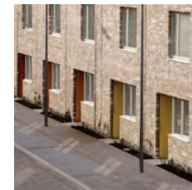
5. Full timber, painted front doors with glazed sidelight in differing colours along the street.
